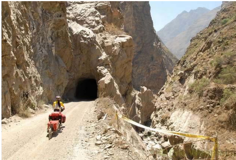
36 tunnels unsecured and also without illumination had to be crossed in the Cañon del Pato
